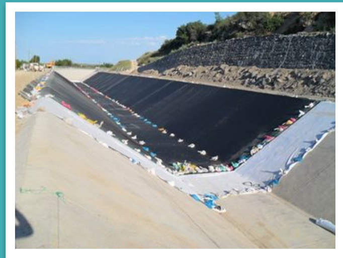
Canal Lining Works
